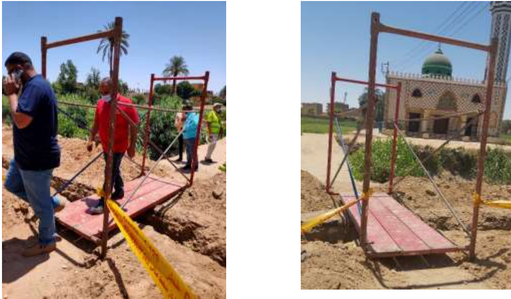
Figure 3-5 Pedestrians safe footbridge
