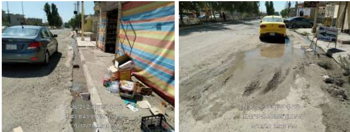
Figure 3-3 The Current Status of the subproject area
