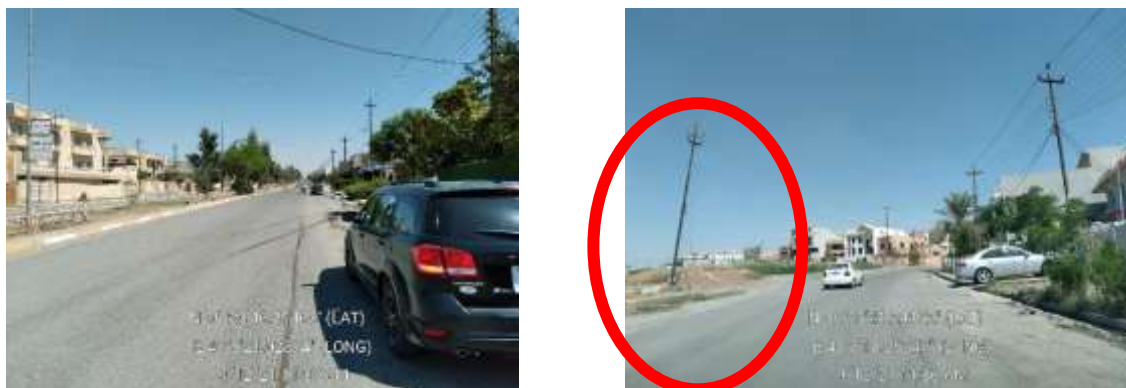
Figure 4-17 Electricity network on the left Bank
