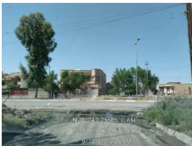
Figure 4-12 Types of residential building
