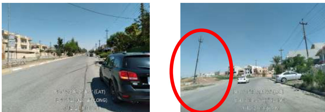
Figure 4-17 Electricity network on the left Bank
