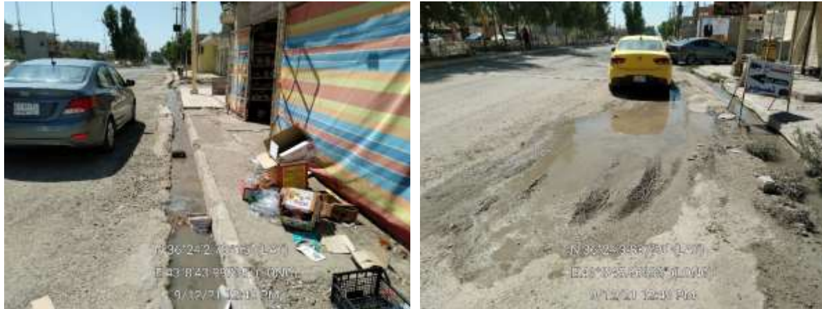
Figure 3-3 The Current Status of the subproject area
